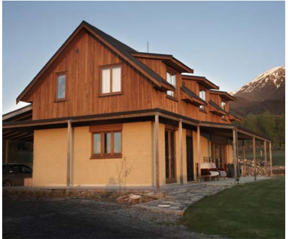
The dwelling is an Adobe ground floor and light timber construction first floor as per NZS 4299.2024. Photo supplied by Verena Maeder of Solid Earth Ltd.
