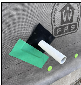
STEP 2: Remove one side of the split backing paper from the ES60 Tape, place the exposed adhesive side onto the FPS® Seal, ensuring equal lengths of ES60 Tape extend beyond each end of the FPS® Seal.
