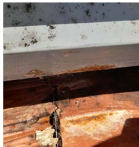
No matter what the substrate, prolonged excessive internal moisture will cause failure of metal cladding
