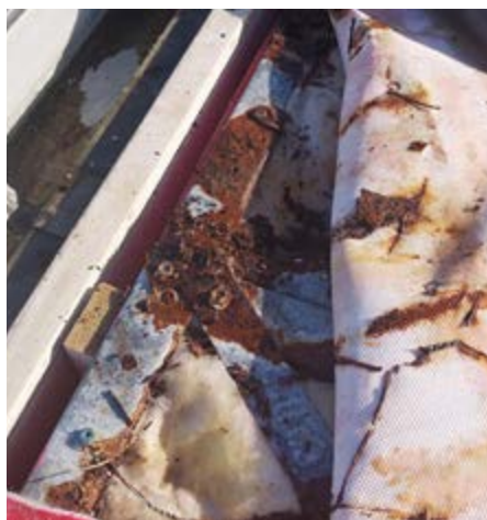
No matter what the substrate, prolonged excessive internal moisture will cause failure of metal cladding
