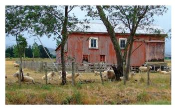
Old woolsheds like this are fire bombs waiting to happen. Without sprinklers, any fire gaining a foothold in such a structure would be unstoppable, fuelled by decades of old grease, oils and dried droppings. Photo: Ross Milller.
