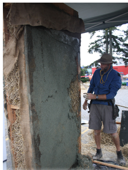
Touching up the plaster after the panel has been raised to the vertical
