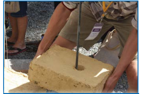
Emplacing a mud brick
