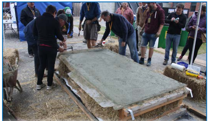
TOB straw panel filled & plastered, awaiting erection
