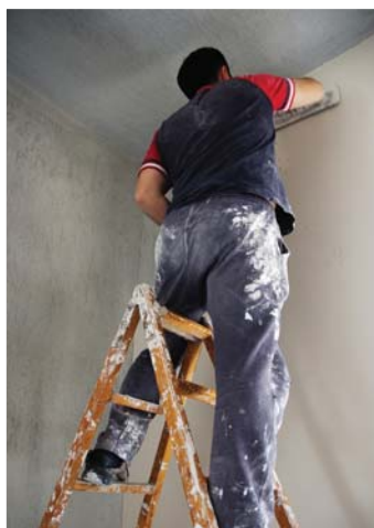
Plastering the board joints in partitions (above) and the junctions of wall and ceiling (left).
