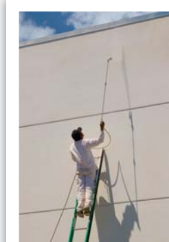
Water or oil based paints applied on pre installed Promat boards.
