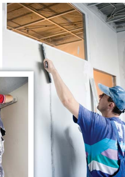
Plastering the board joints in partitions (above) and the junctions of wall and ceiling (left).
