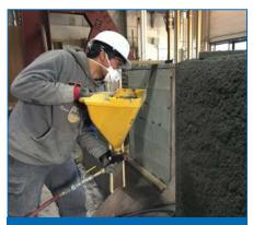
Plastering a wall with seismic-resistant concrete (UBC)
